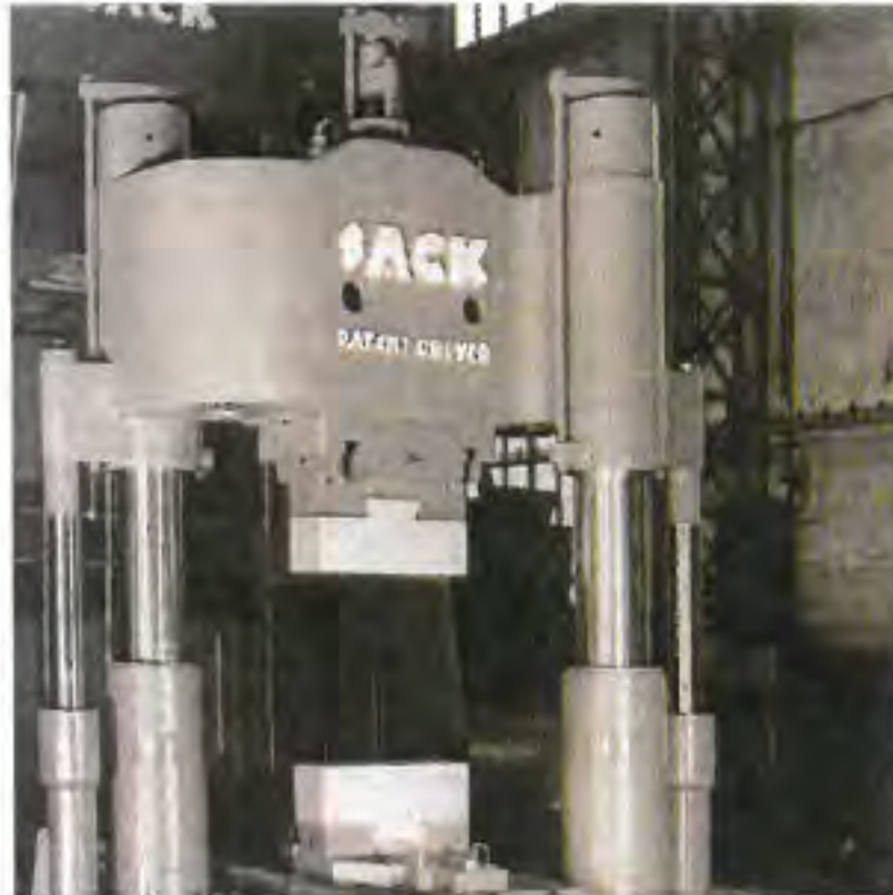
1956: The first open die forging press with 10 MN press force built under the direction of Hans-Joachim Pahnke. A pull-down design with Z-shaped cross-heads.
